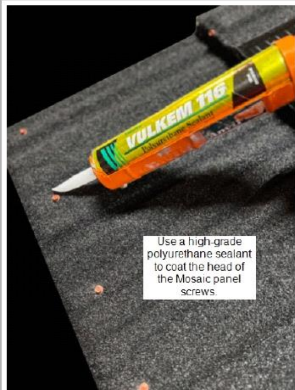
Polyurethane sealant applied over screw head.
