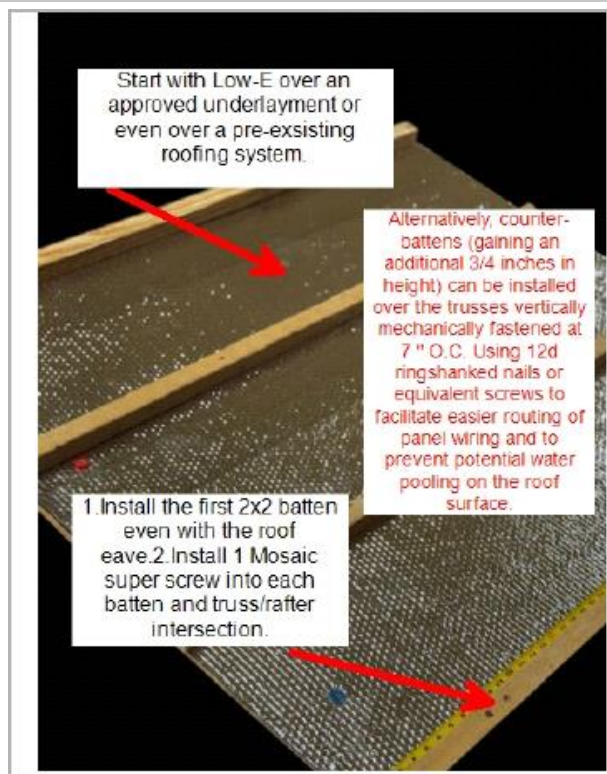
Eave starter batten and initial low-E/underlayment condition.
