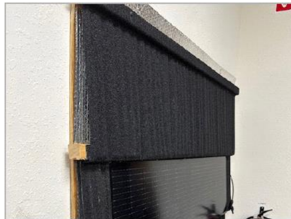
Finished Powerhouse display - side elevation.
