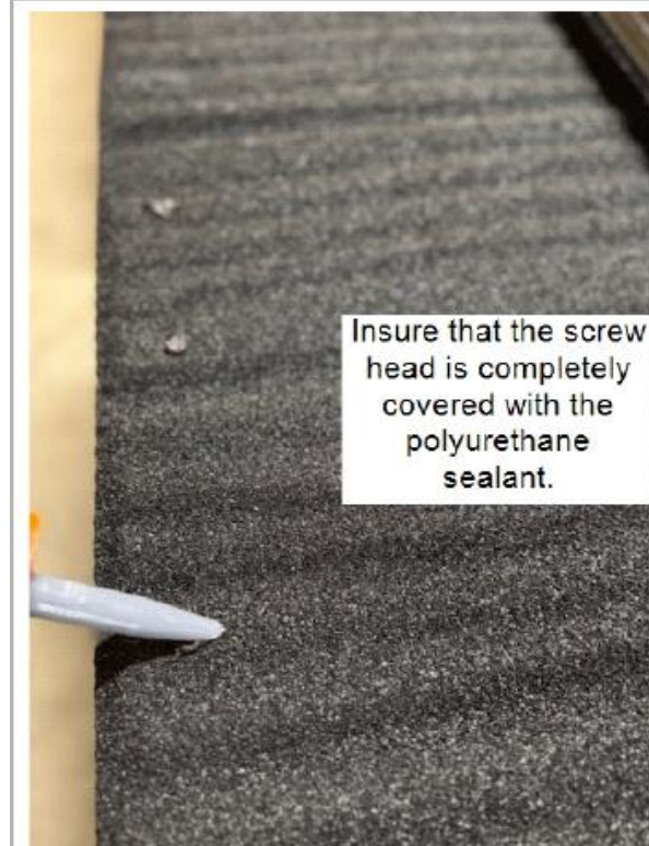
Screw head fully covered with sealant.
